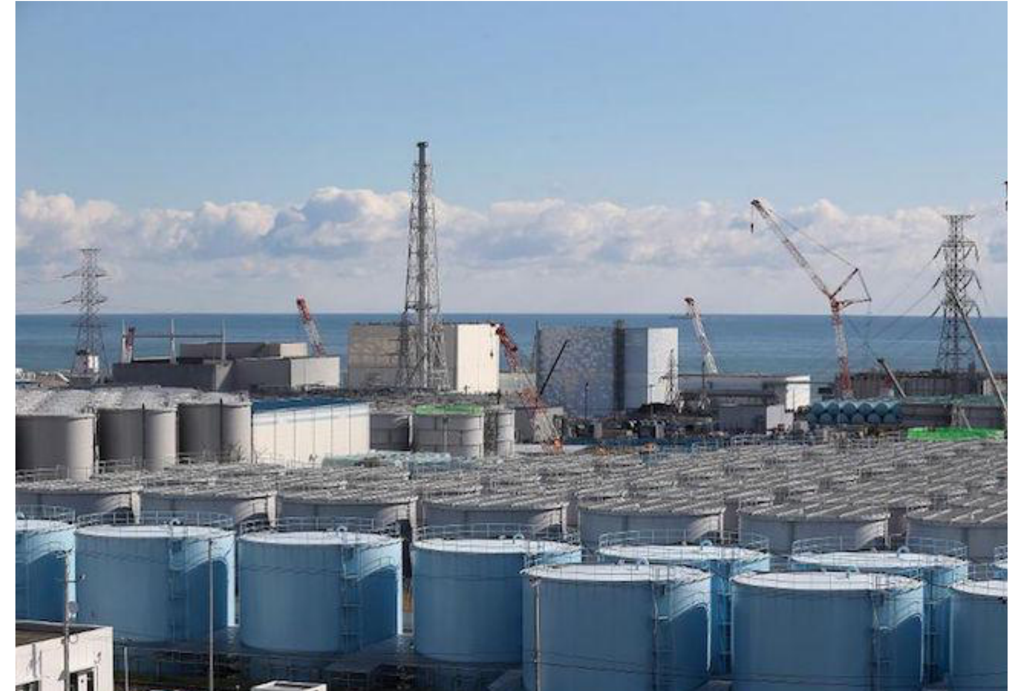
Tanks storing treated groundwater flowing through destroyed fission power plants at Fukushima
