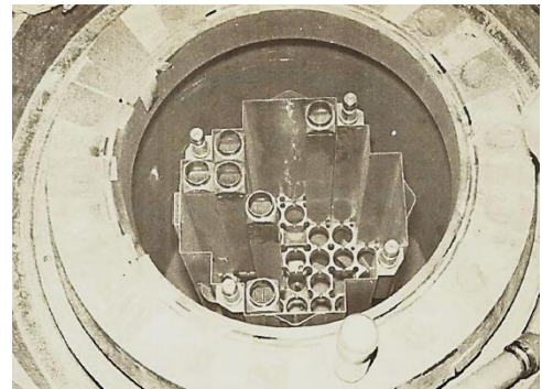
Figure 3. Six training fuel elements loaded into PM-2A reactor during testing at Dunkirk, May 1960 [10]
